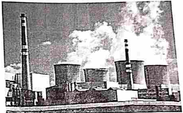
Figure 9.17 : An Atomic Power Generation Plant
